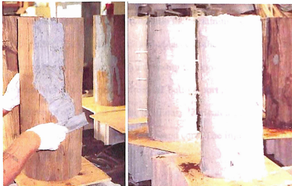
FIG. 3.5. Application of Epoxy Mortar Coating on Laboratory Repaired Timber Piles
