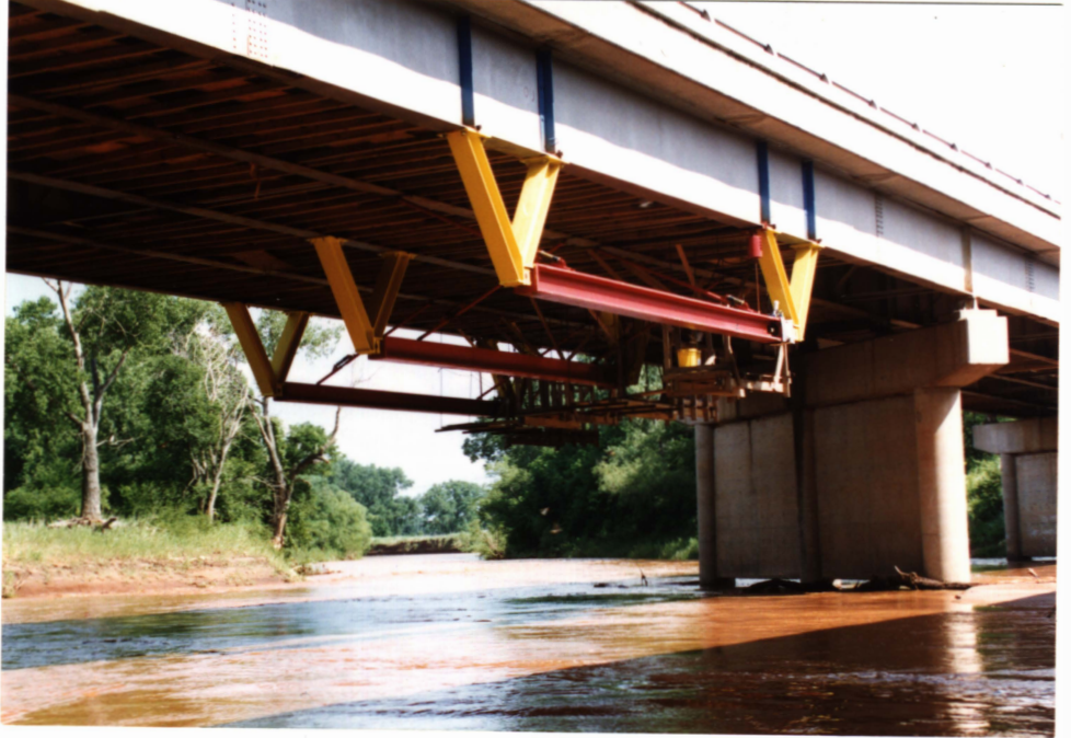
Photo 1: The I-35 Walnut Creek Bridge with SAVA System Attached
