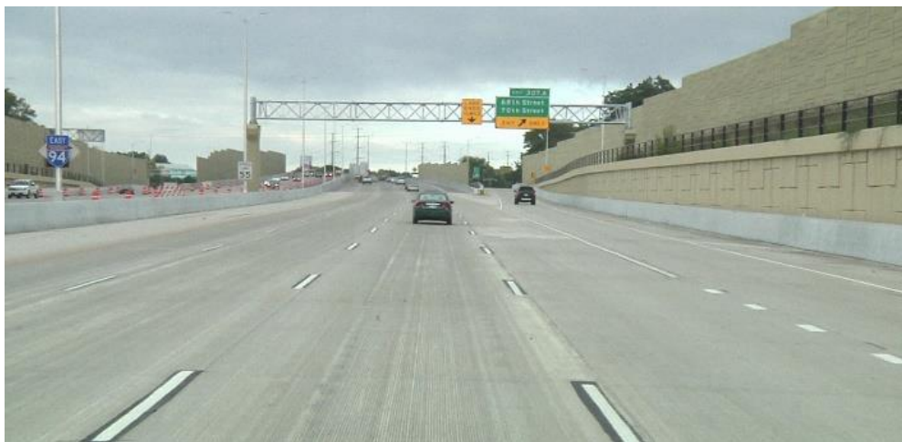
(f) Grooved Rigid Pavement (WI-I94)
