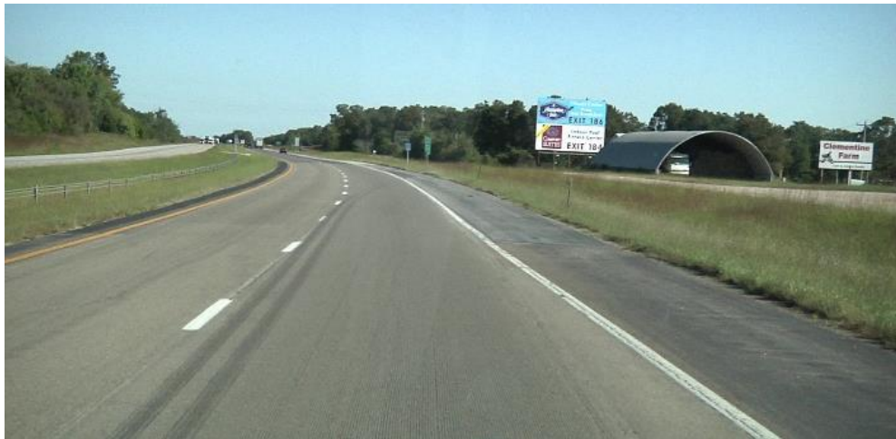
(e) Grooved Flexible Pavement (MO-I44)
