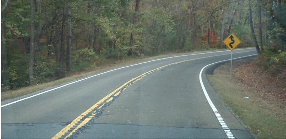
(a) HFST Pavement (GA-140)
