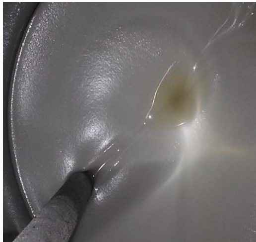
Top view of the reservoir
