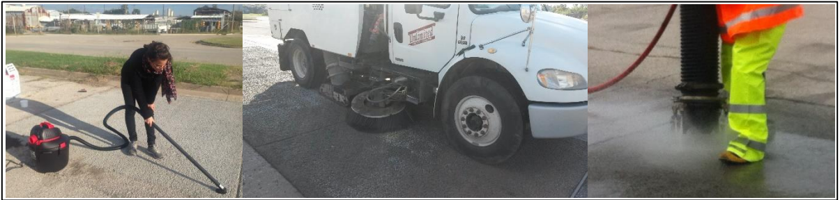
Figure 4.2. Pervious concrete cleaning methods. Left: hand vacuuming; Center: street sweeper; Right: Vactor truck
