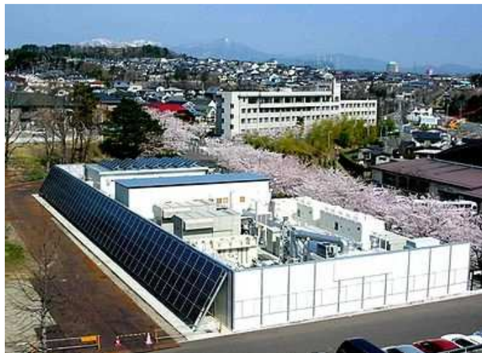
Figure 1.2. Microgrid at Fukushi, Japan
