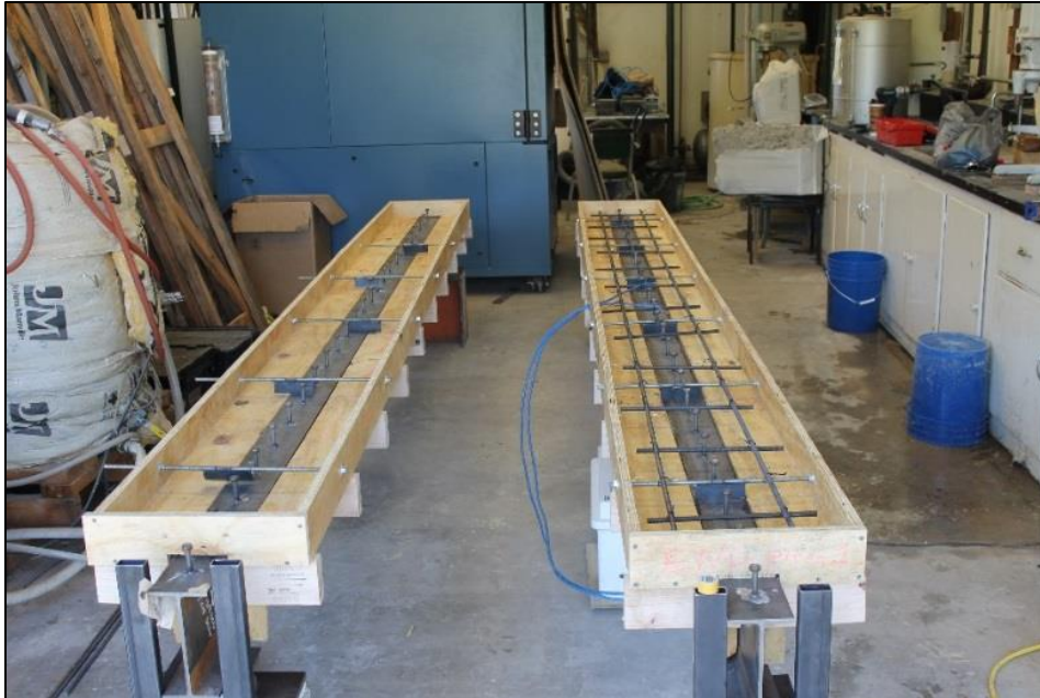
Figure 4: Formwork for concrete decks that were cast-in-place atop W8x15 steel girders.
