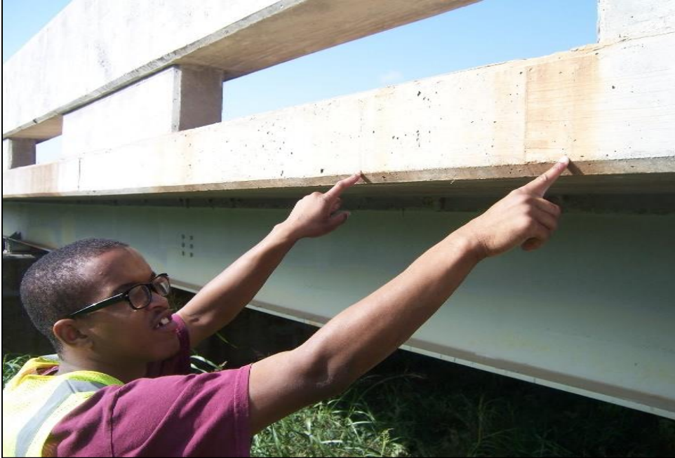
Figure 29: Identifying crack locations on SH 14 Eagle Chief Creek “A” in Woods County
