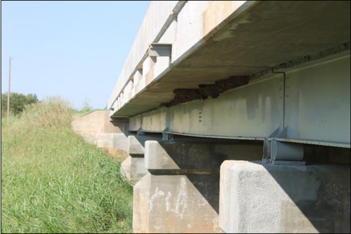
Figure 60: SH 14 bridge over Eagle Chief Creek in Woods County
