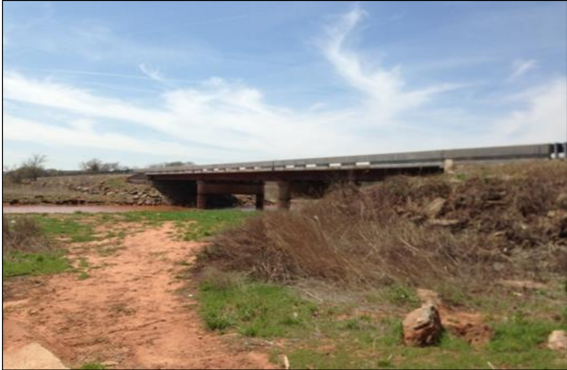
Figure 55: SH 86 over Stillwater Creek in Paying County
