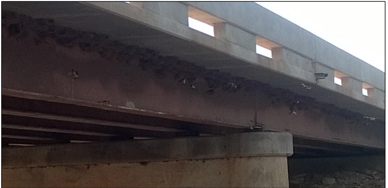
Figure 28: Observing the superstructure and sub-structure of US 286 in Payne County
