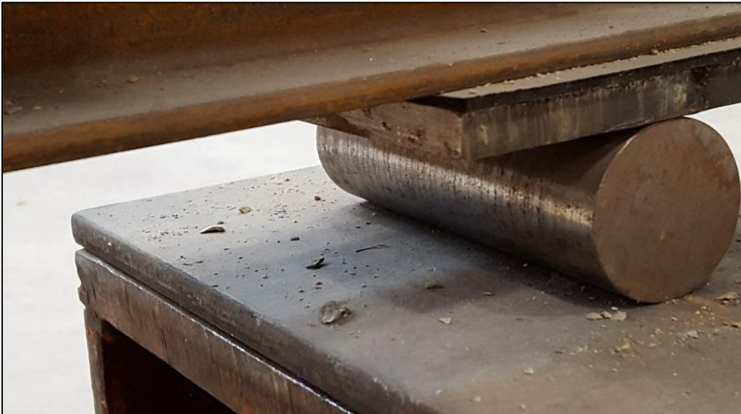
Figure 7: Roller support on the prototype beams
