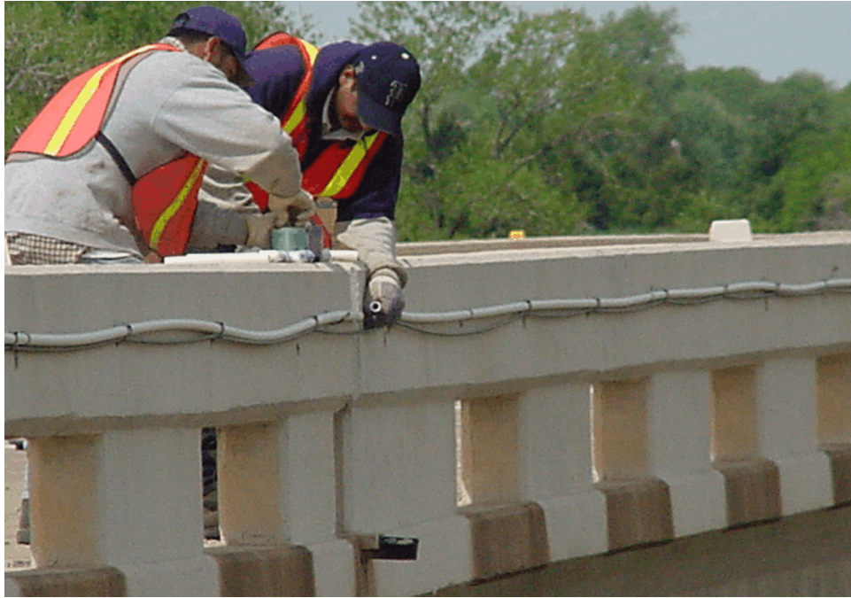
Figure 15. PVC Supply Lines
