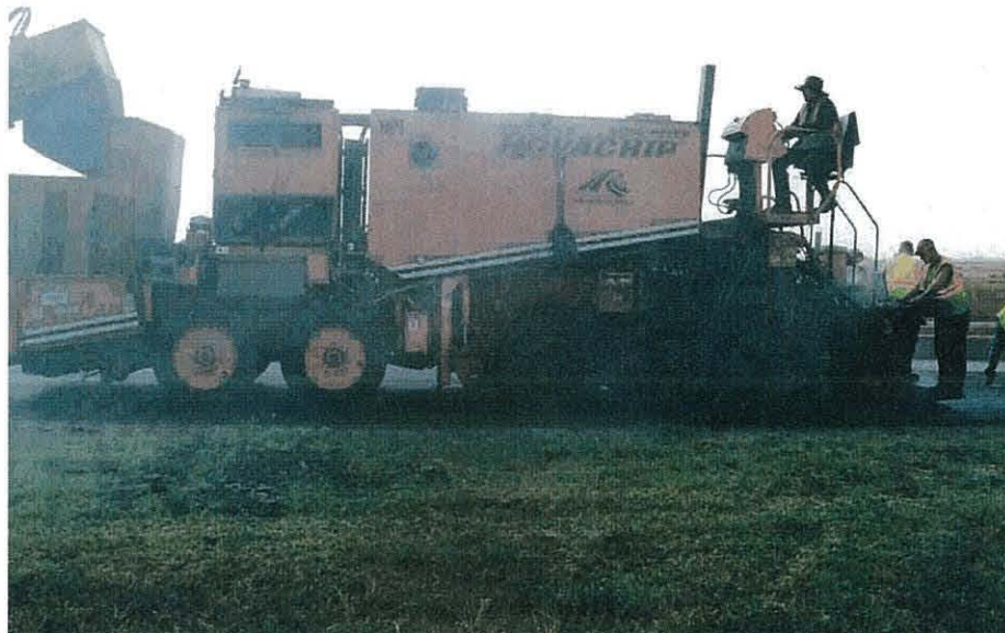
Figure 4. A NovaChip laydown machine.
