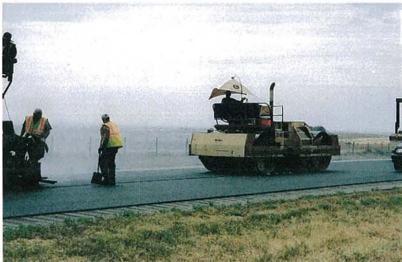
Figure 7. Connell Construction Company rolls Novachip.
