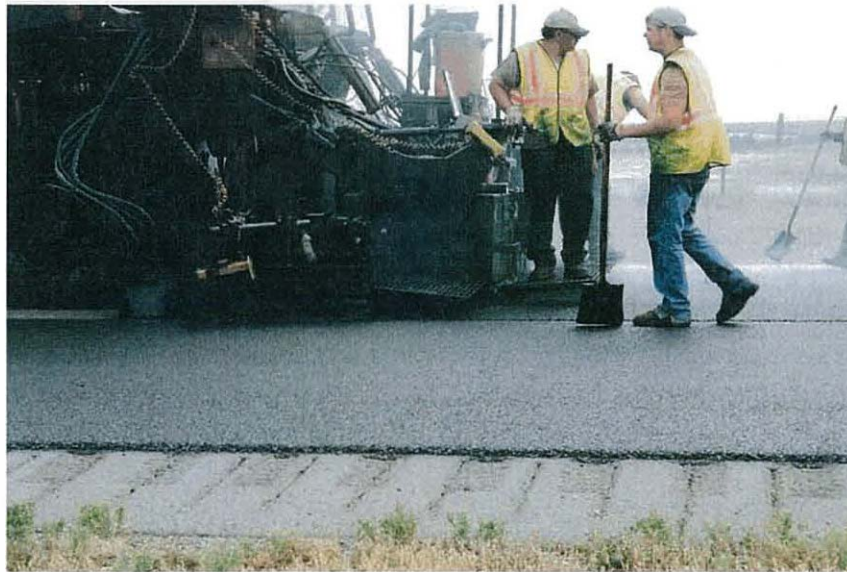
Figure 6. Placing a NovaChip mat.
