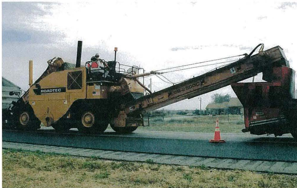
Figure 3. An asphalt transfer machine mixing NovaChip and placing it into the hopper.
