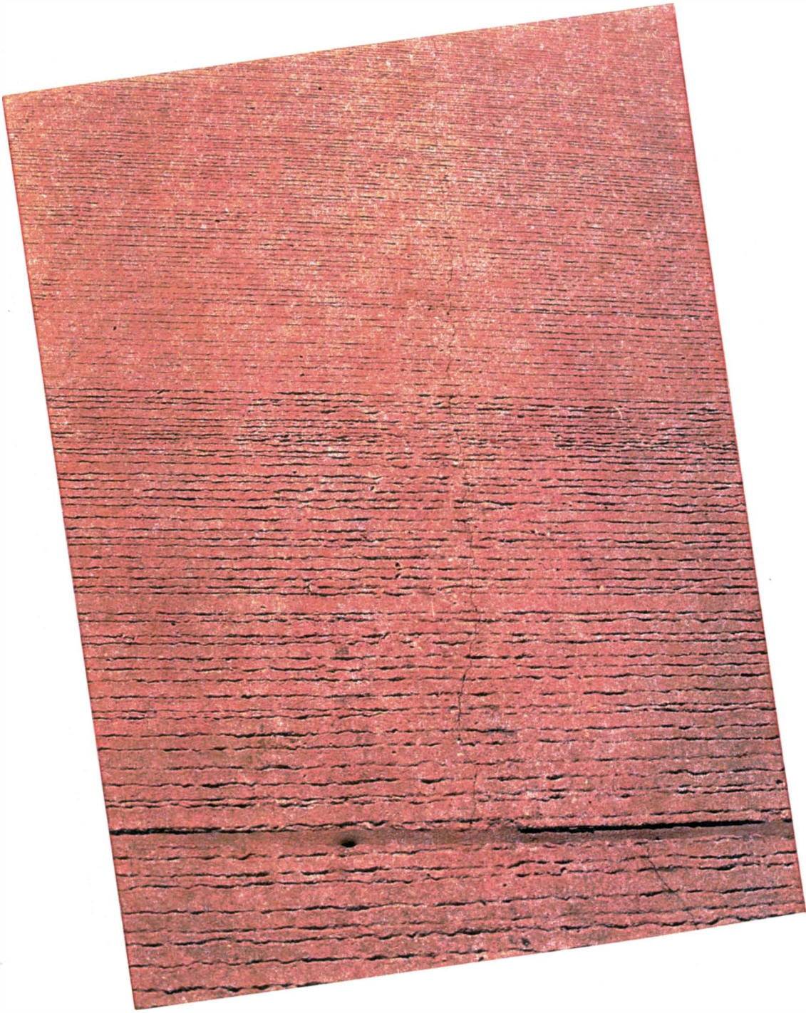
Figure 2 Longitudinal Cracking
