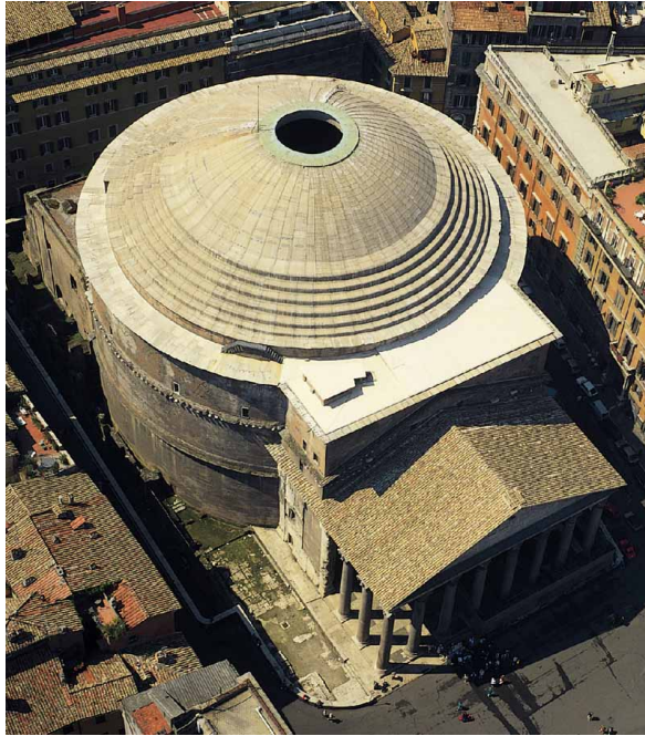
Figure 1: Aerial view of Pantheon in Rome (Architexts 2016)
