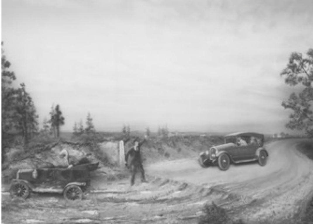
Figure 2.8: “Mud at the State Line” shows how good roads is not a local issue, but a national issue because of the interstate traffic. Source: NARA-II 119-M-1A-27.
