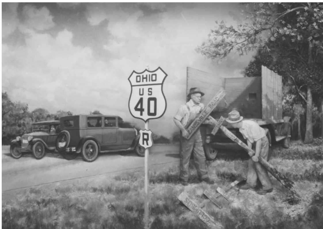
Figure 2.7: The BPR released this photo of how they replaced inconsistent signage with those of a national standard, an aesthetic representation of national uniformity. Source: NARA-II: 119-M-1A-45.
