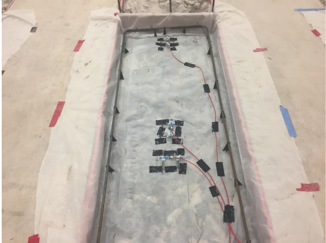
Figure 17, Instrumented Slab with No. 5 Reinforcing bar
