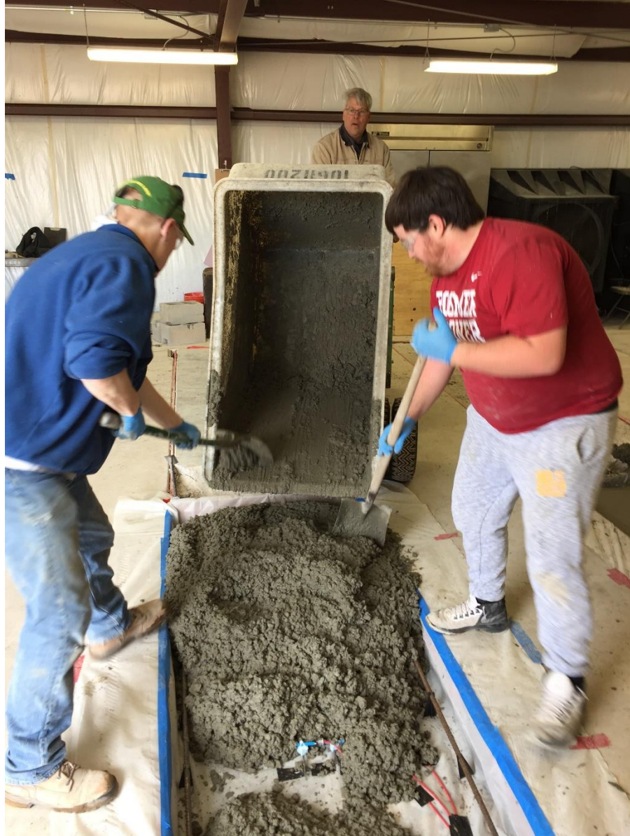
Figure 30, Placing Concrete in Forms from Concrete Buggy
