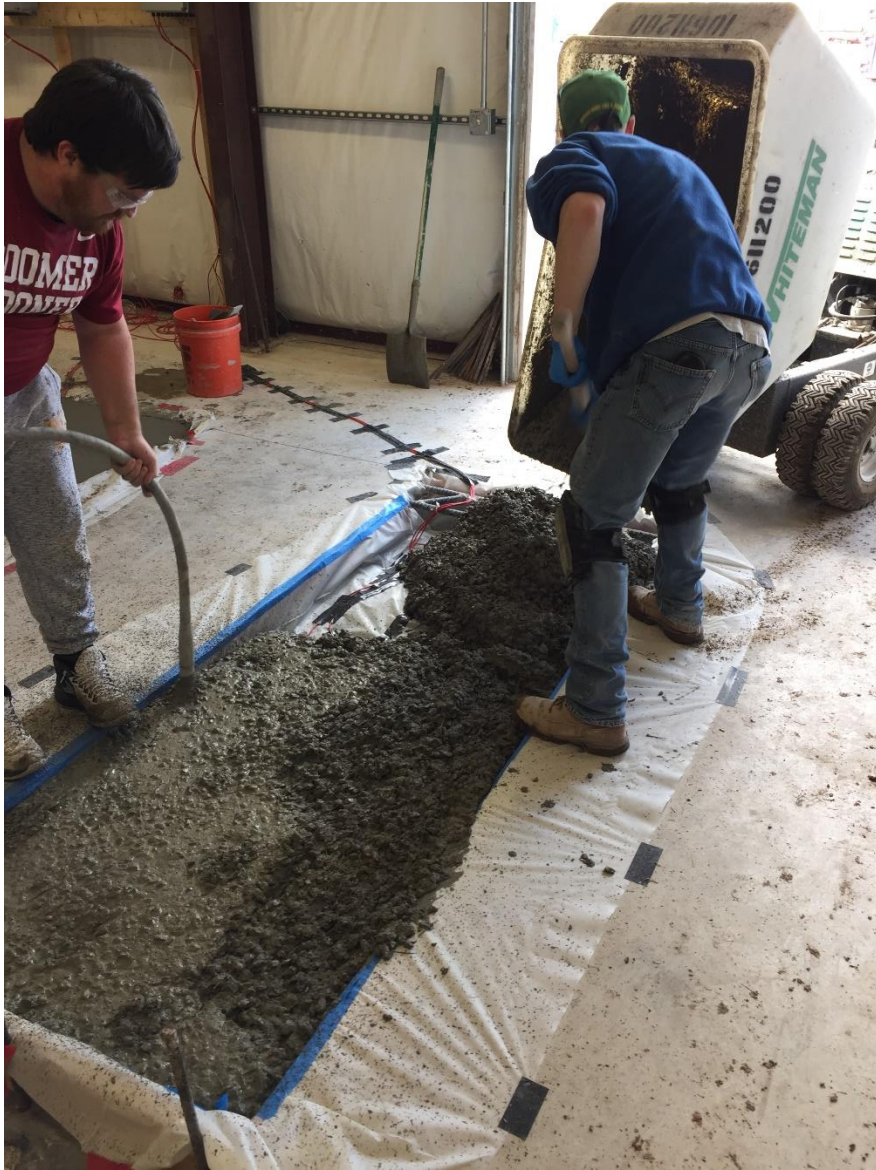
Figure 31, Vibrating Rod Consolidating Slabs
