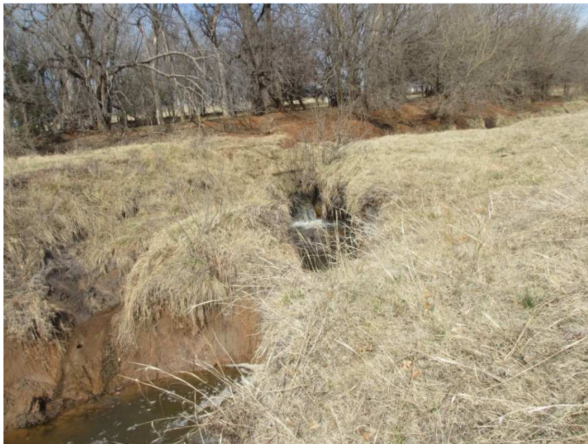
Figure B4. Cross-sectional survey and ground based photograph for site FM2 XSEC3.
