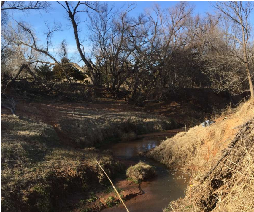
Figure B14. Cross-sectional survey and ground based photograph for site WC3.
