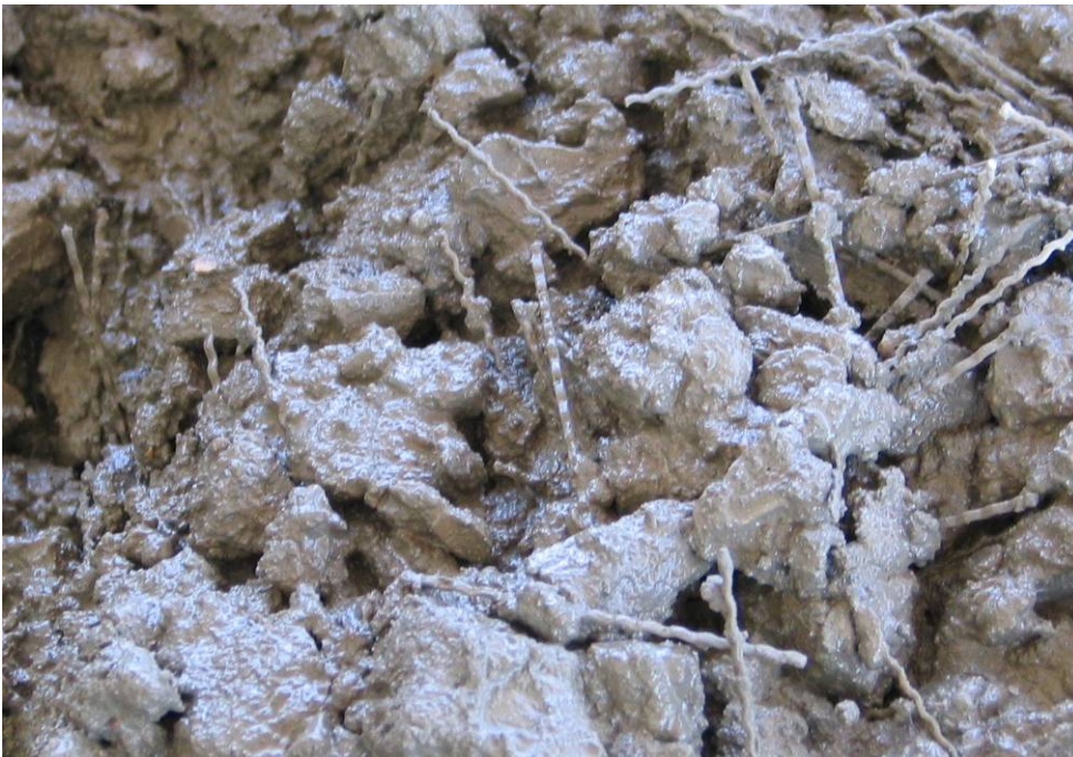
Figure 33: Concrete mixture with high dosage of HPP fibers
