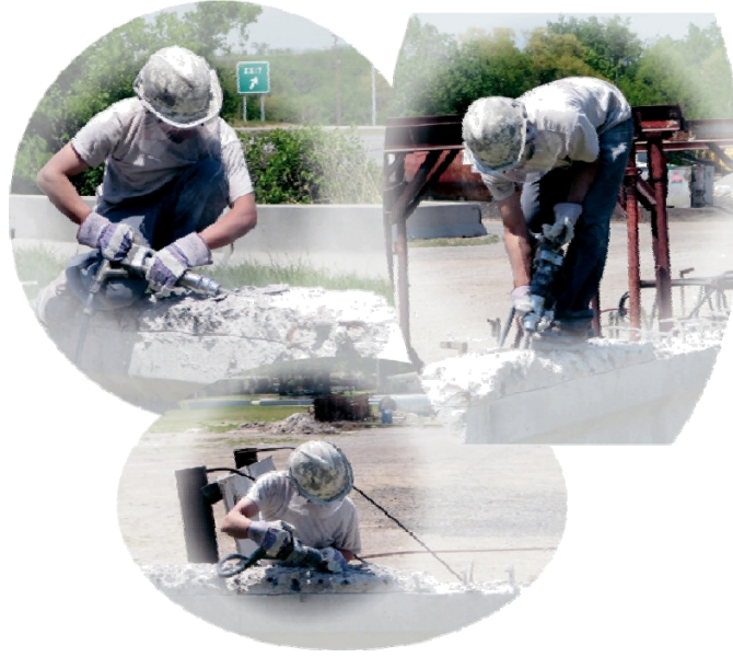
Figure 5: Augustine, a Concrete Services Corporation employee, removing remaining slab on April 21, 2006
