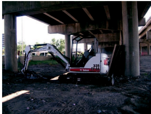
Figure 4: Track hoe used to demolish the girder from the I-244 Bridge.
