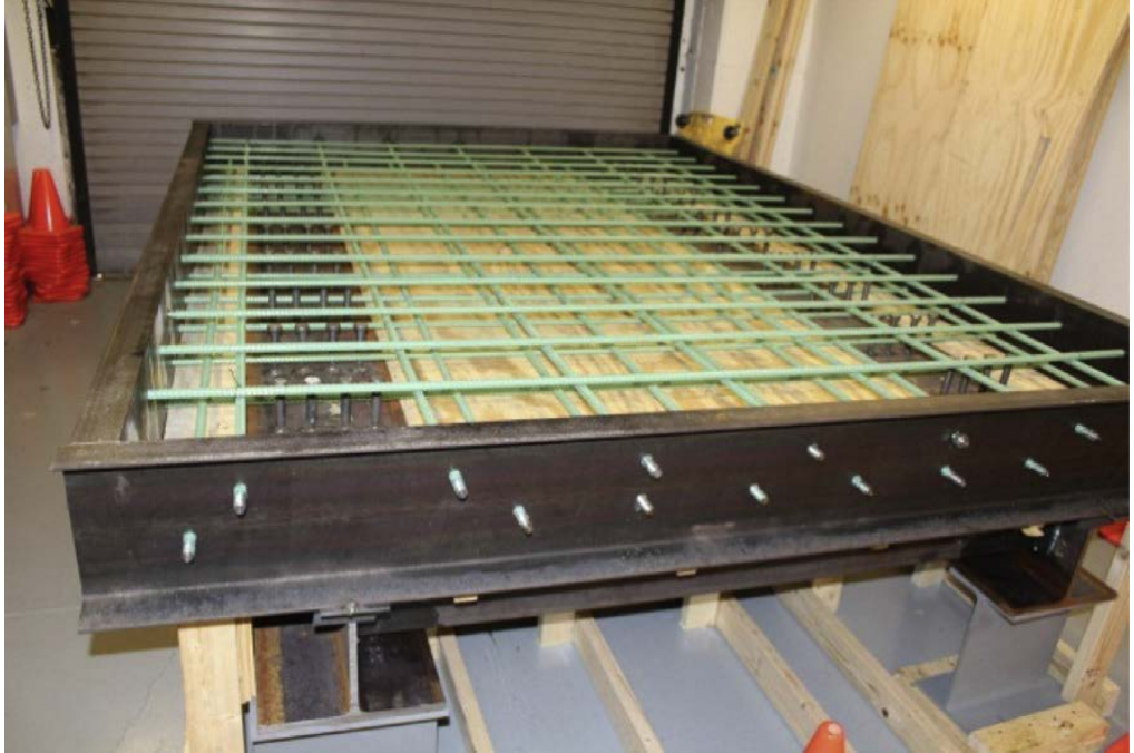
Figure 6: Test Setup for Experimental Bridge Deck (Richardson et al., 2014)
