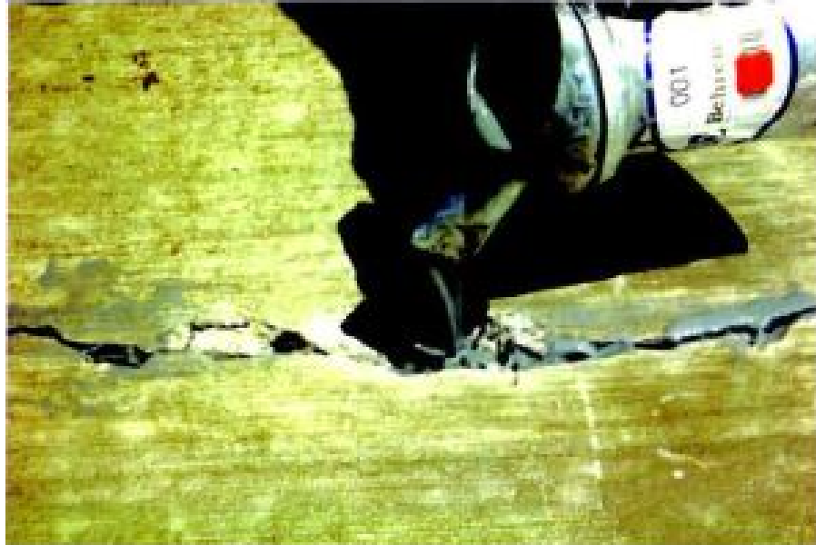
Figure 4: Transverse Crack Repair at Greater Rockford Airport (Chusid, 2006)
