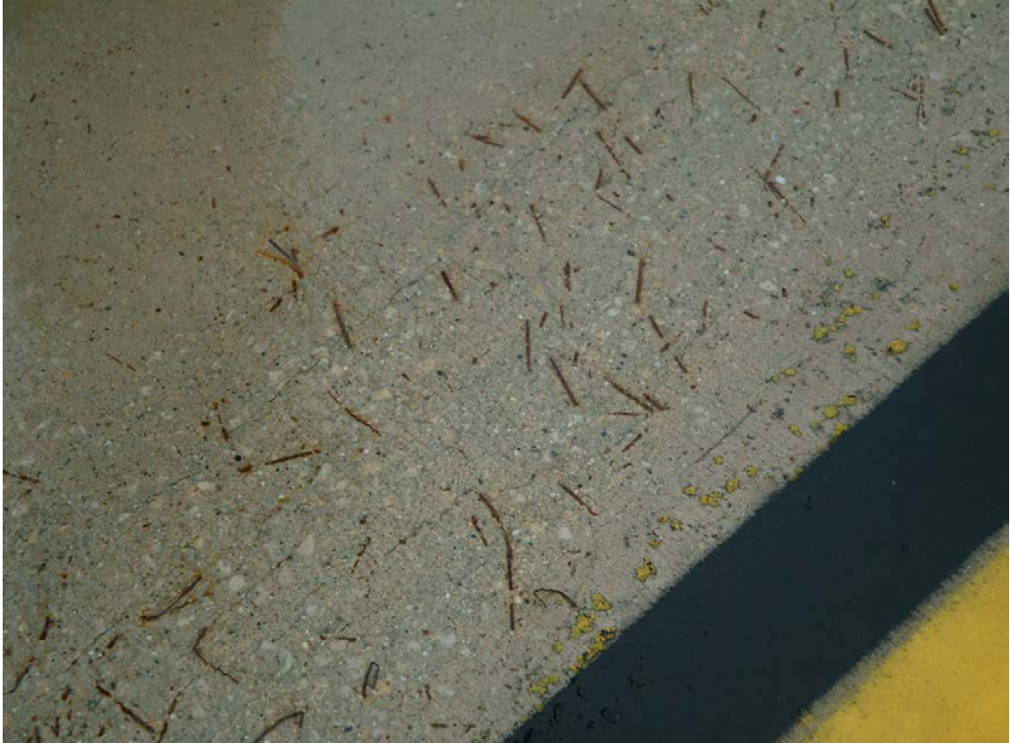
Figure 1: Airport Runway Slab with Steel Fiber Reinforcement at Greater Rockford Airport (Ramseyer, 2018)
