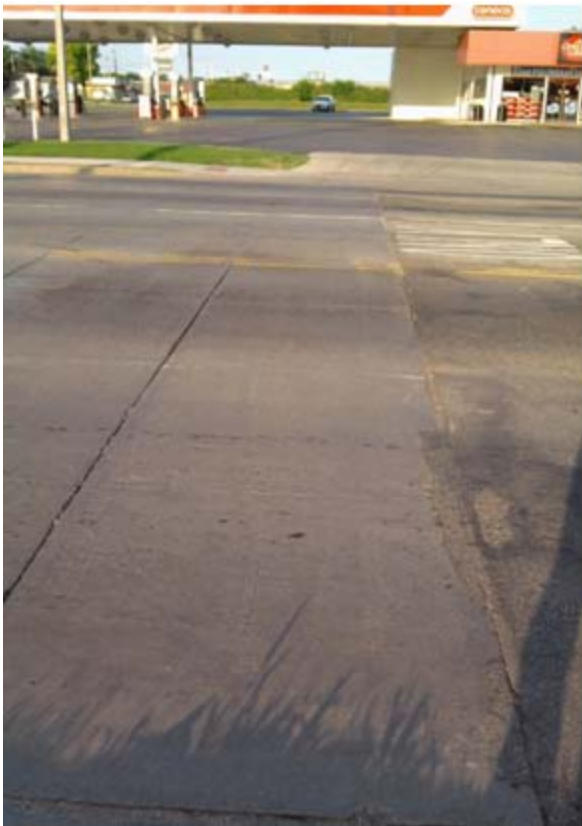
Figure 2.32 - Approach on US 177 from south showing excellent condition of initial panels.
