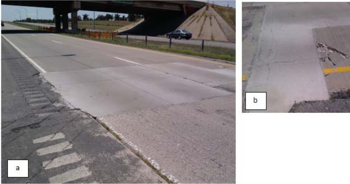
Figure 2.15 – Photo a shows the repaired panels at the north end of the overlay. Photo b shows a cracked panel at the west end of the overlay.
