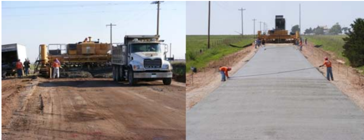
Figure 2.48 - Photos show the construction of the overlay.
