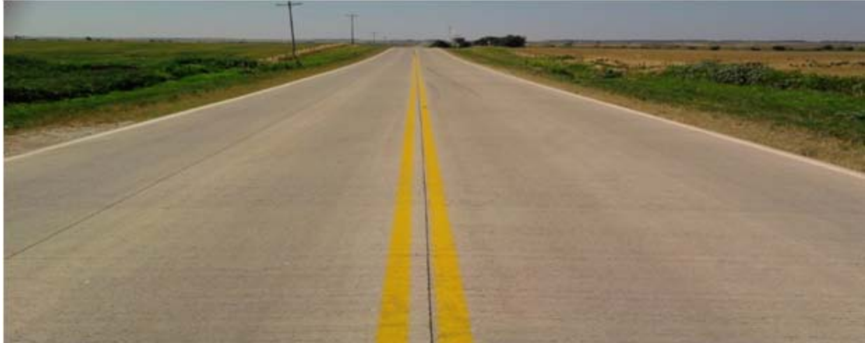
Figure 2.53 - Photo showing the excellent condition of the overlay.
