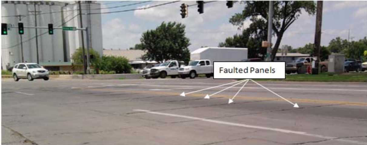
Figure 2.41 - Photo showing faulting as seen from east end of the intersection. A repetitive noise was heard from the tires of the vehicles when they passed on the faulted panels.
