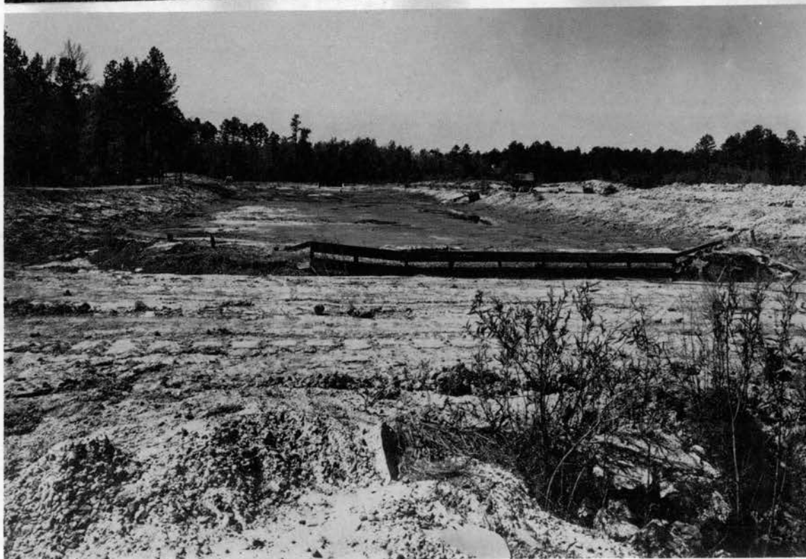
Plate I Settling Basin: Upper in operation, lower drained in preparation for dredging.
