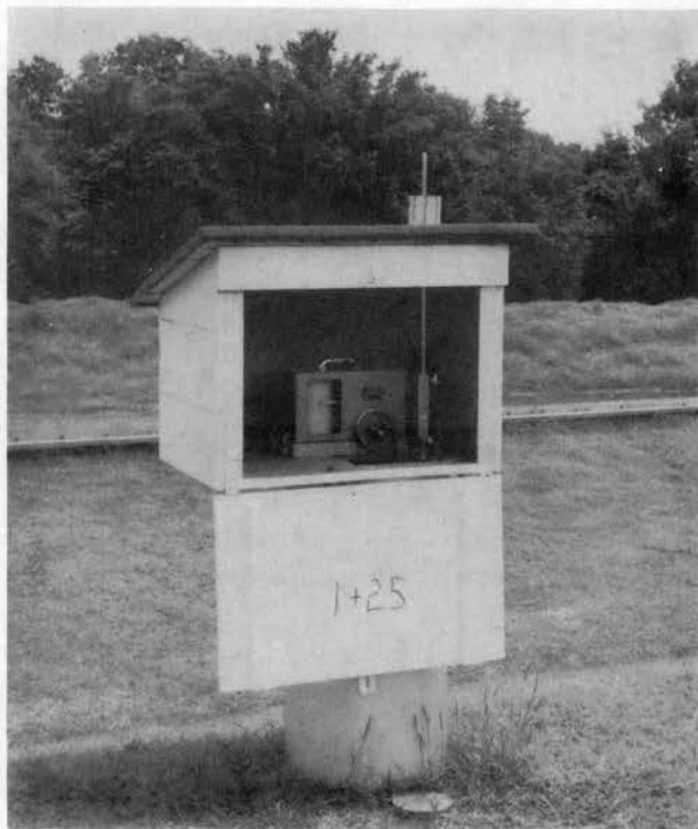
Figure 12. Gage Well and Equipment
