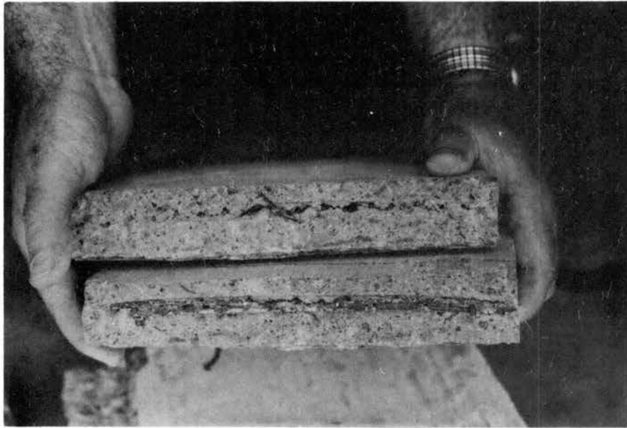
Figure 29. Failure Section of Panel 14-1, Showing Void Along Crosswire at Failure.
