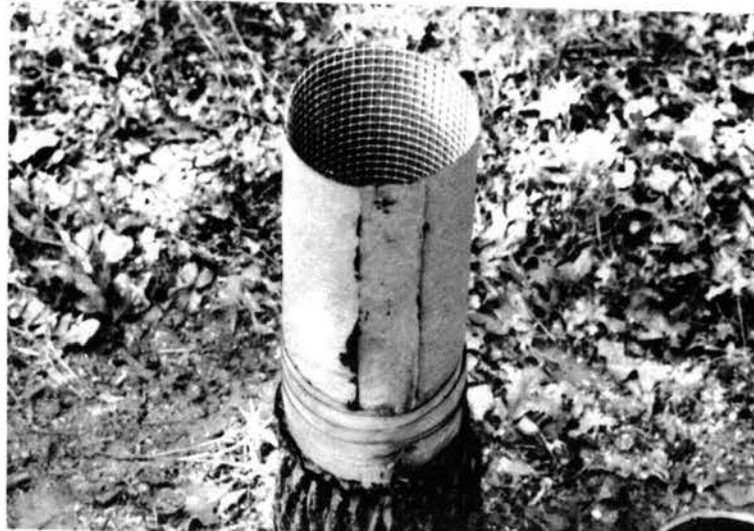
Figure 6. Collar Sealed and Reinforced
