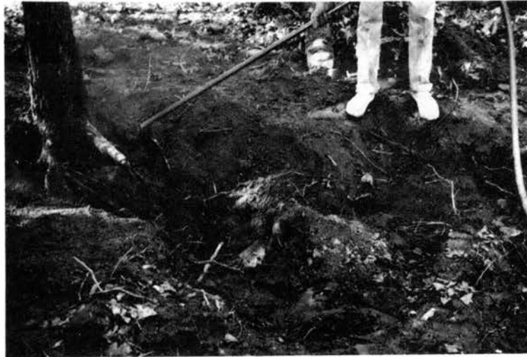
Figure 24. The Air Excavation Tools in Use
