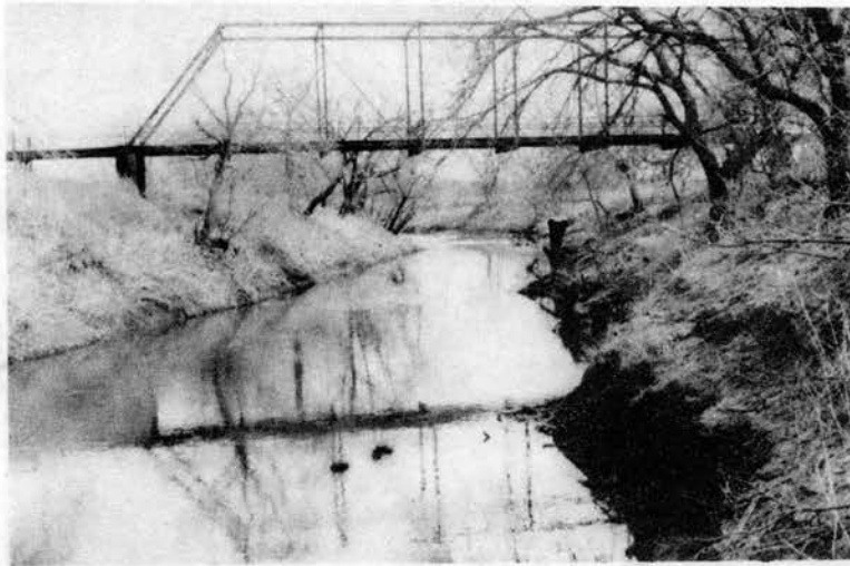
Figure 6. Location of gaging station on Washita River near Chickasha (4th St.). The arrow points to a limb which caused reverse flow along the right bank in the cable suspension section.
