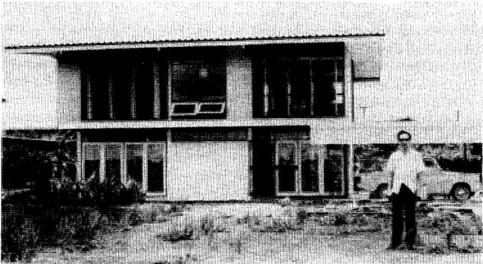
Modern Compound Housing, South Elevation
