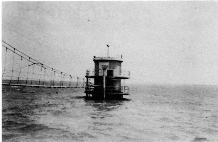
Figure 5. Intake Tower Instrument Site.
