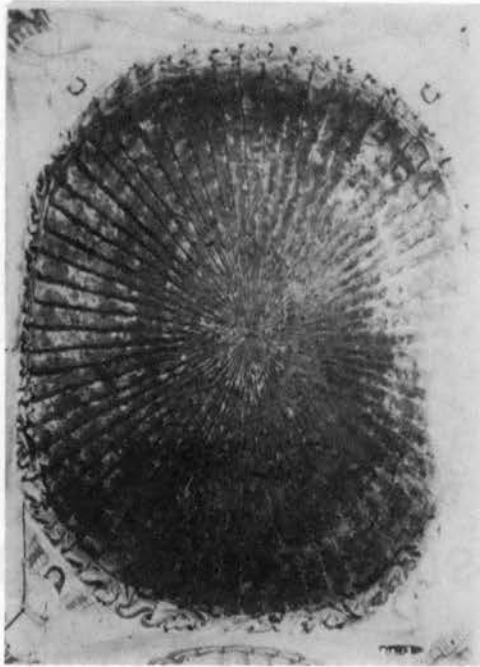
Figure 28. Vault Over the Second Bay in the Nave.
