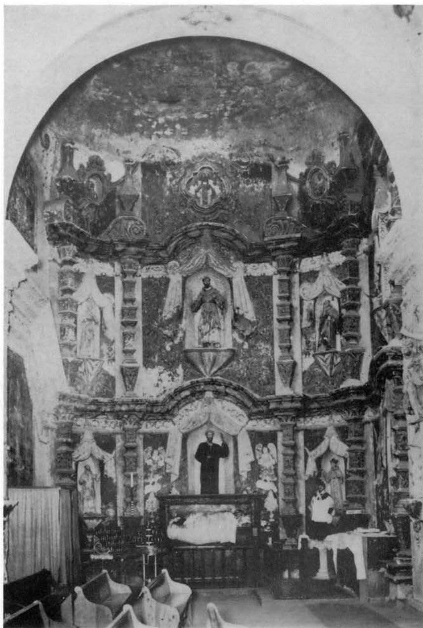
Figure 31. Main Altar, The West Transept, Chapel of the Suffering Savior. East Elevation.
