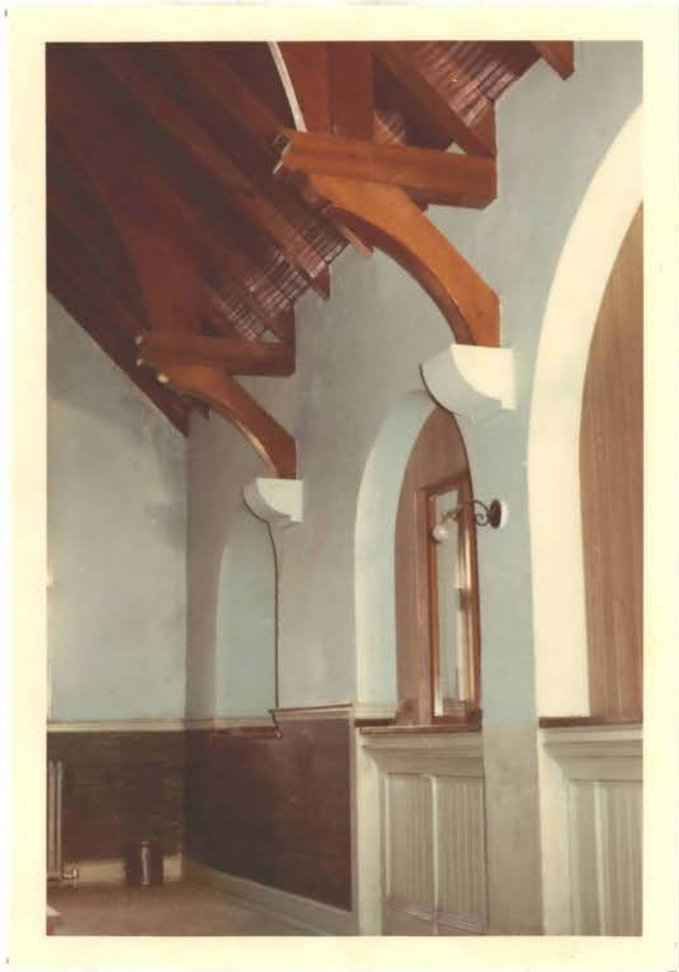
Figure 25. Hammerbeam, Santa Fe Railway Station Shawnee, Oklahoma
