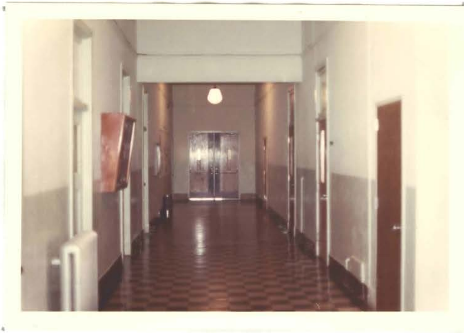
Figure 18. Original First Floor Corridor, St. Gregory's College
