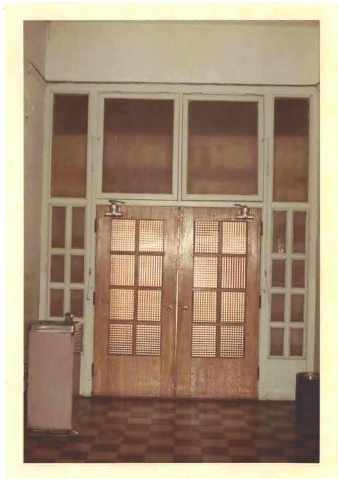
Figure 21. Doorway, East View, First Floor Corridor, St. Gregory's College
