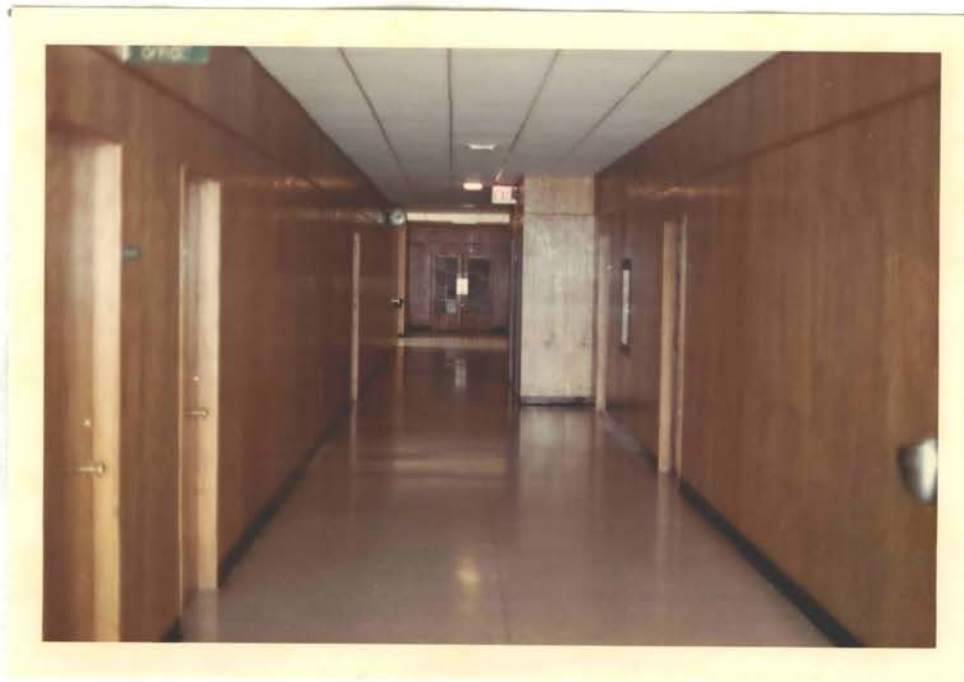
Figure 19. Remodeled First Floor Corridor
