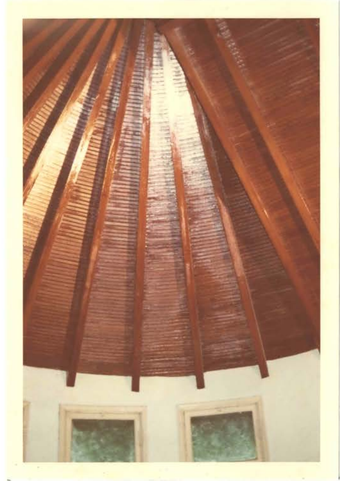
Figure 24. Conical Ceiling, Santa Fe Railway Station, Shawnee, Oklahoma
