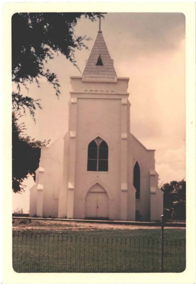
Figure 7. Exterior View, Sacred Heart Church
