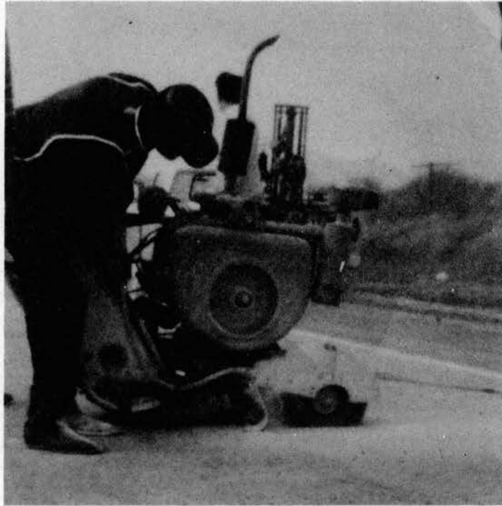
Figure 3.5. Workman Using Pavement Saw to Cut a Channel in PCC Pavement
