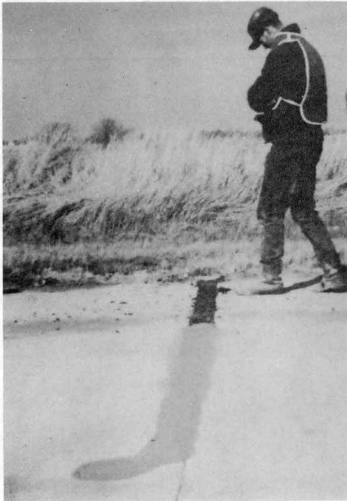
Figure 3.8. Channel After Patching
