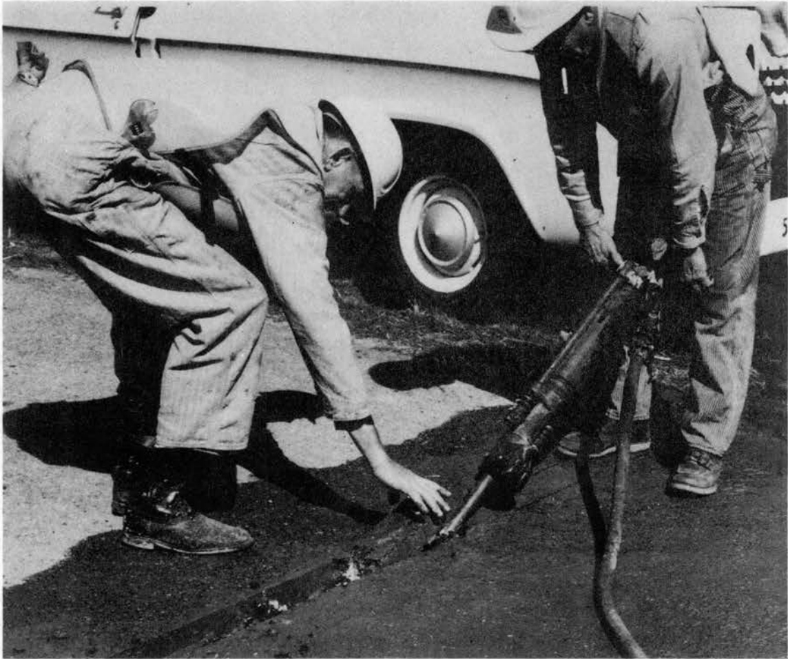
Figure 3.6. Workmen Removing Material from Channel
