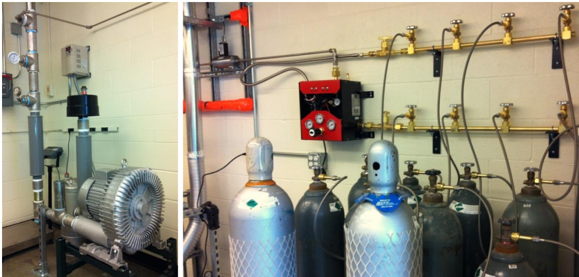
Figure 5.9. Gas injection section
