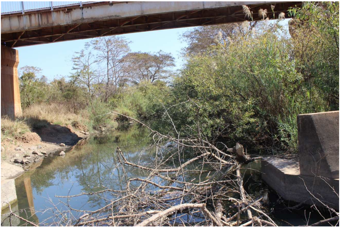
Photo 30. Bridge over the Kananapa River near sampling location.
