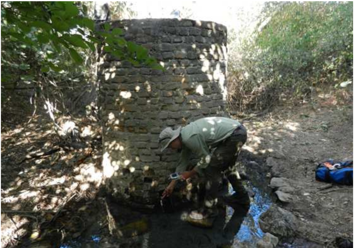
Photo 86. Circular brick structure built around the spring at West Acres Farm.
