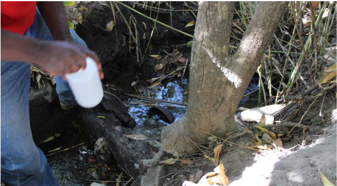
Photo 12. The concrete collection area just prior to diversion to the pipe
