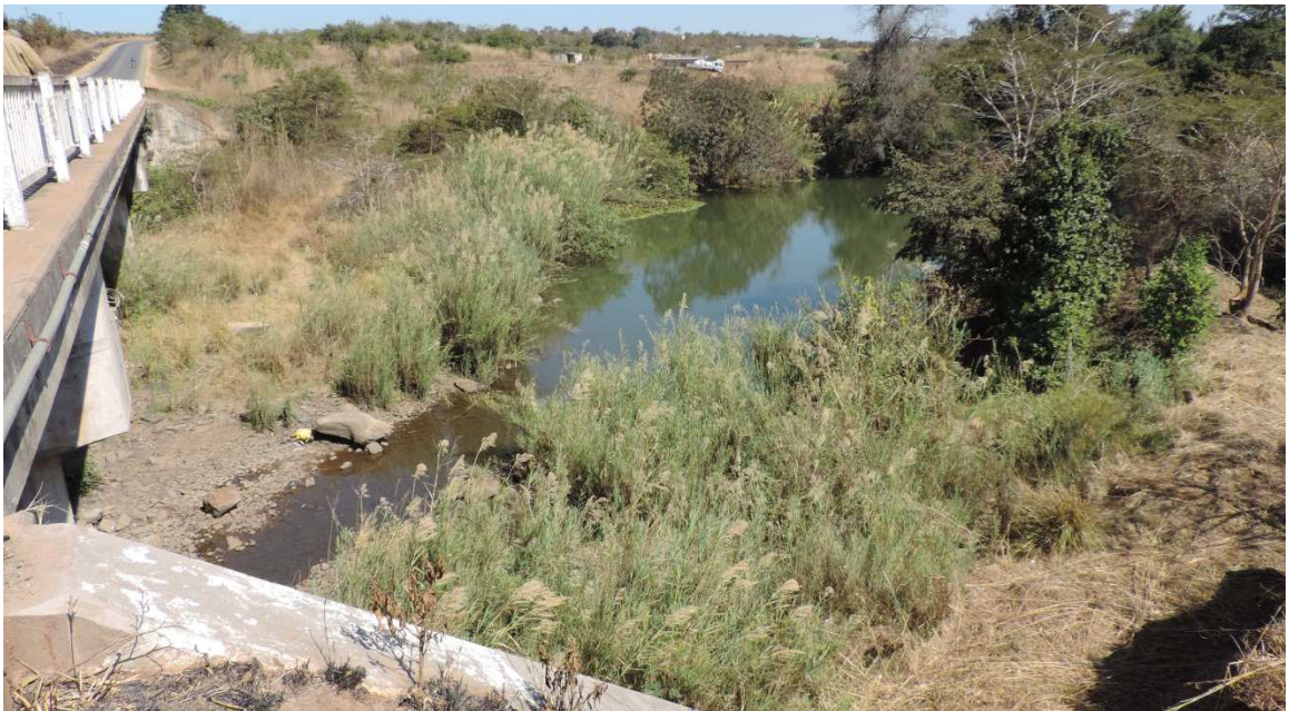
Photo 18. Chongwe River looking west on the north side of the bridge.
