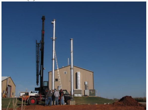
(f) Columns in place
