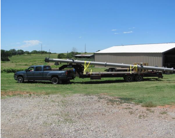
(a) Column delivery to ASU site
