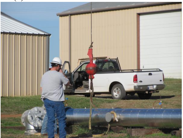
(e) Lifting trunnions in use
