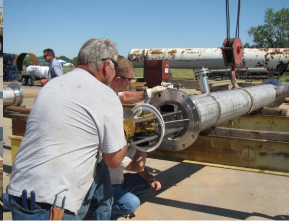
(b) Tray installation in beer column
