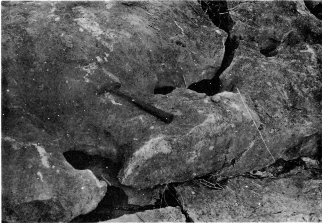
Figure 9.--Cavernous weathering of limestone in the Hughes Creek Shale at Phillips Lake spillway.
