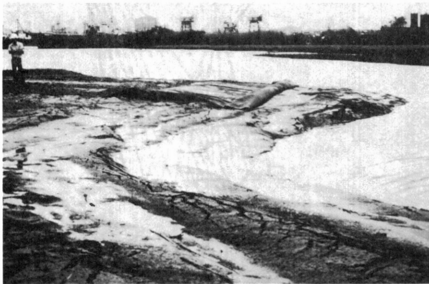
Figure 52. Polyfilter X Fabric Being Rolled onto Advancing Mud Wave Caused by Fill Material and Fabric Displacement of Soft Foundation Materials
