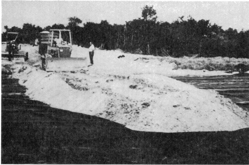
Figure 47. Construction of Parallel Haul Road at Toe of Embankment
