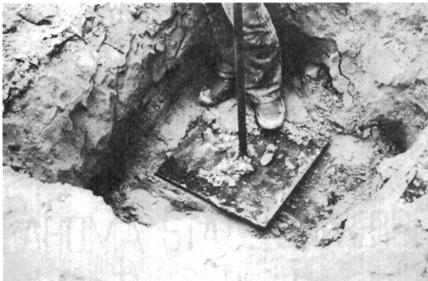
Figure 65. Settlement Plate Being Installed on Fabric
