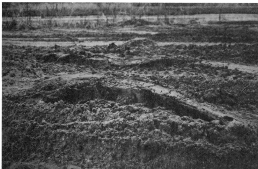
Figure 50. Mud Ways Breaking through Sand Working Table from too Many Passes by Dozer in Spreading Material
