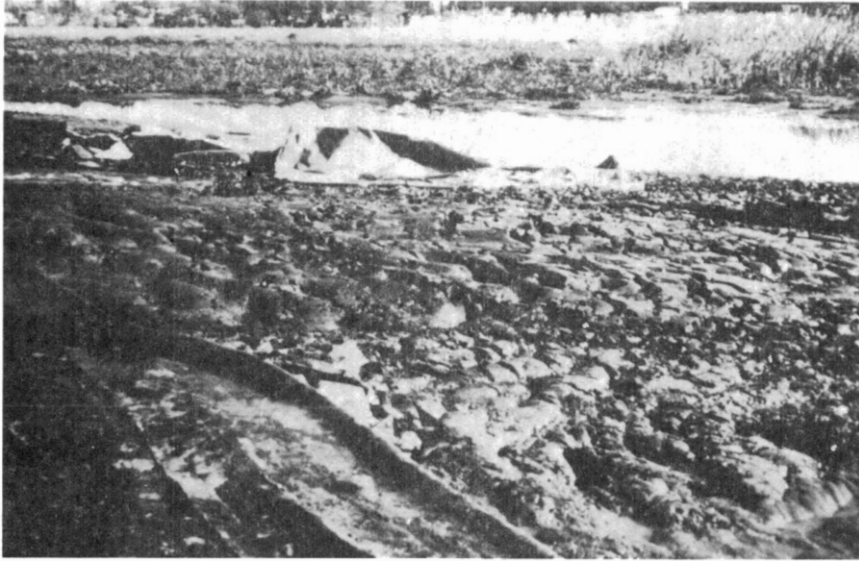
Figure 54. Nicolon 66475 Fabric after Placement and Folding Back for Sewing on Advancing Mud Wave
