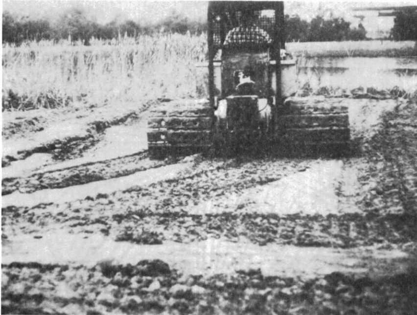
Figure 49. Dozer Advancing Sand Working Table Toward Pinto Pass Channel
