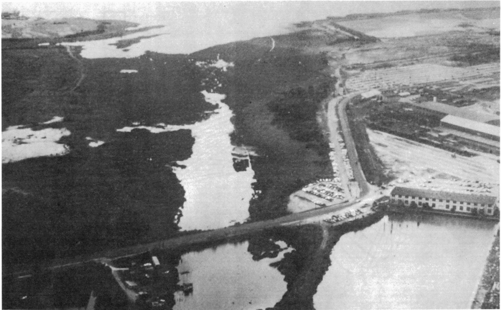
Figure 2. Aerial View of Pinto Pass Looking East to West. Embankment Test Section was Constructed Across Pinto Pass at About Top Quarter Point of the Photograph
