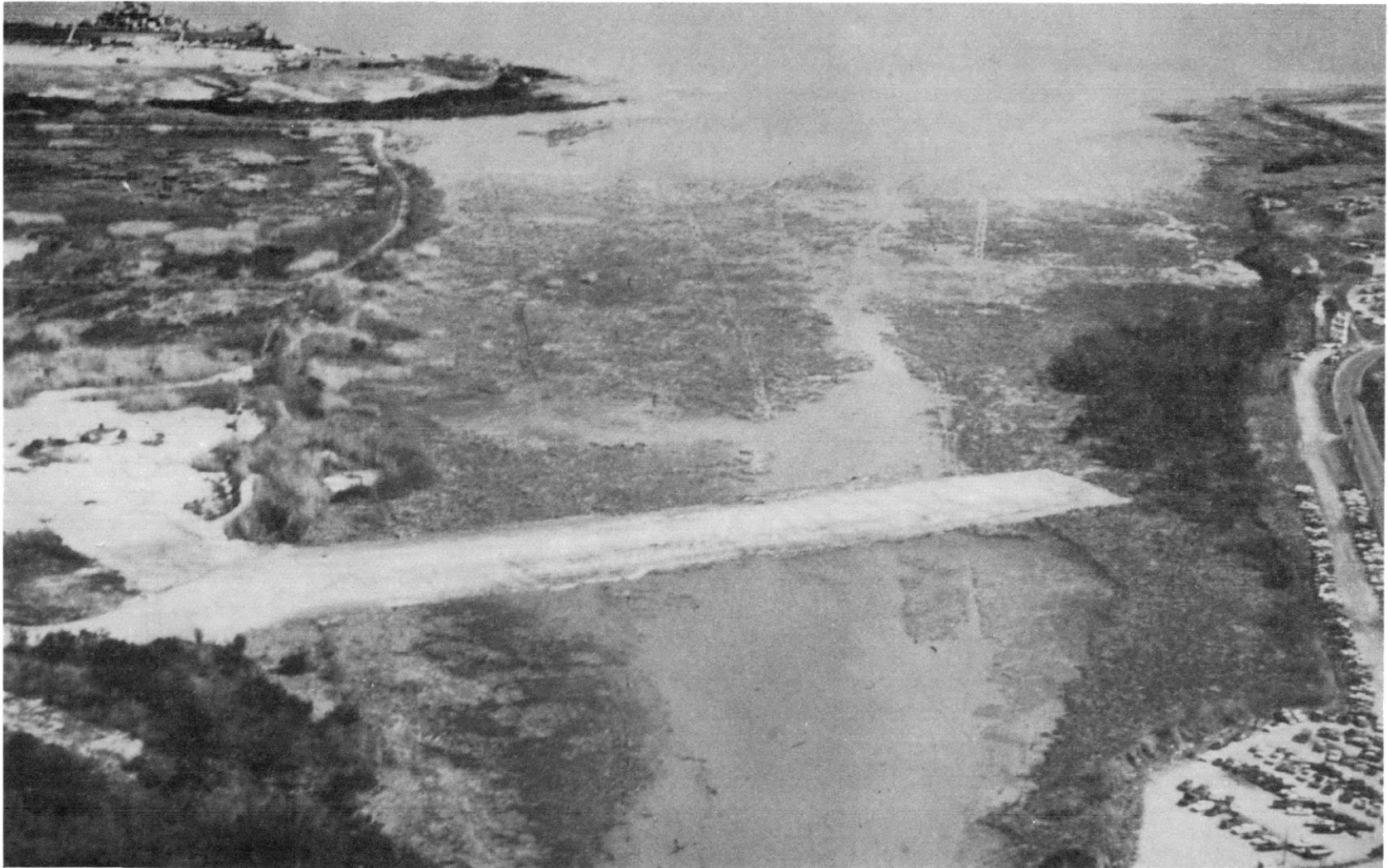
.. Figure 66. Fabric-reinforced Embankment Test Section Completed Across Pinto Pass
