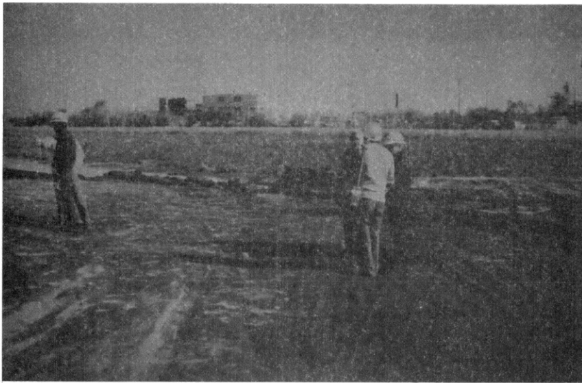
Figure 62. Nicolon 66475 Fabric, Placed Over Soft Foundation Material, Supporting Men
