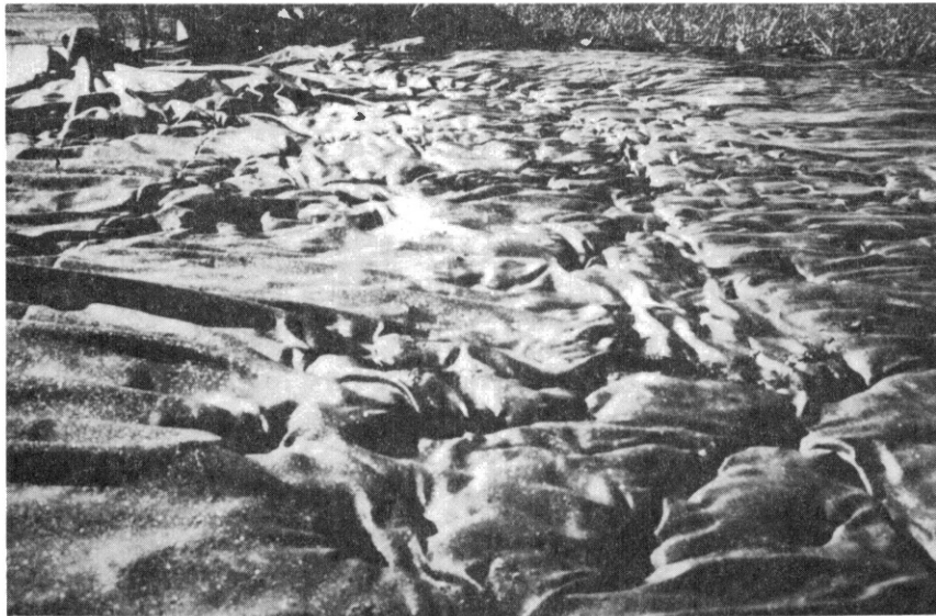
Figure 60. Footprints in Fabric Laid onto Advancing Mud Wave
