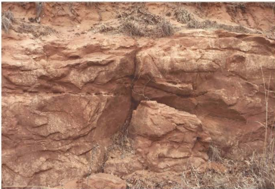
Figure 21. Mass wasting along fractures in sandstone
