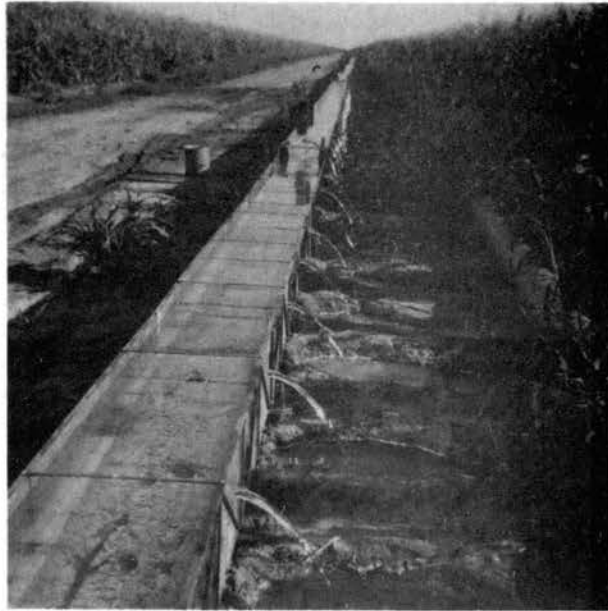
Figure 13. Field Set-Up of Irrigation System
