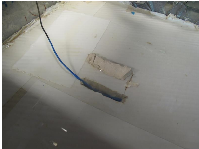
Figure 3-19. Placement of a Pore Pressure Transducer inside Soft Clay
