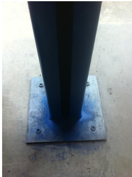
Figure 3.5: Base support for vertical beam
