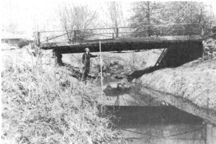
b. Looking Upstream From 9th Avenue Culvert
