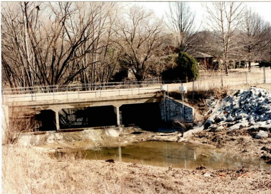
Figure 7. NE Bridge Locality with Rain Gauge
