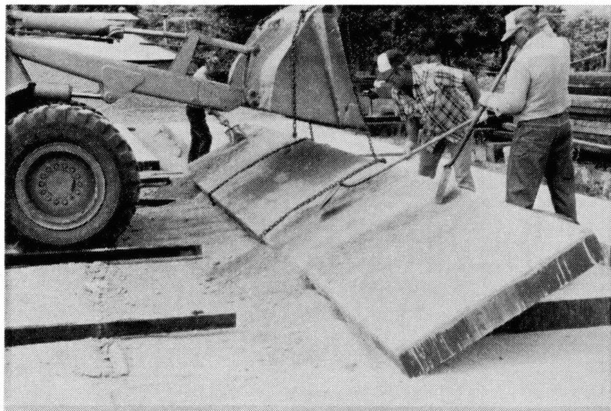
Figure 26. Removing Rock Screenings by Scraping with Shovels
