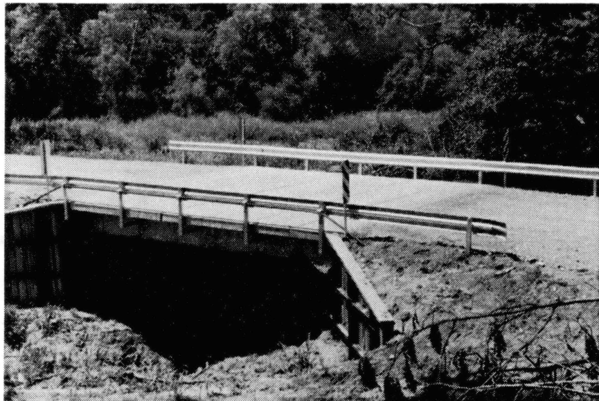
Figure 45. Demonstration Bridge as Viewed from the Northeast
