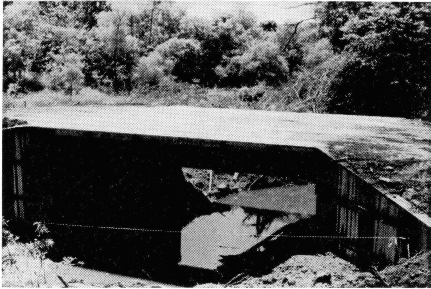
Figure 42. Demonstration Bridge After Twelve Days of Construction
