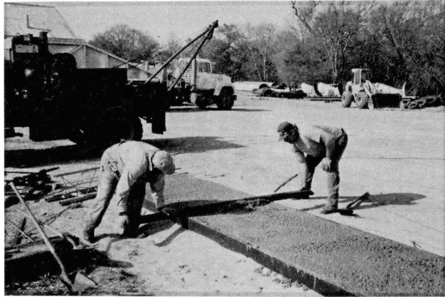
Figure 20. Screeding and Finishing with a 2 x 4 in. Board
