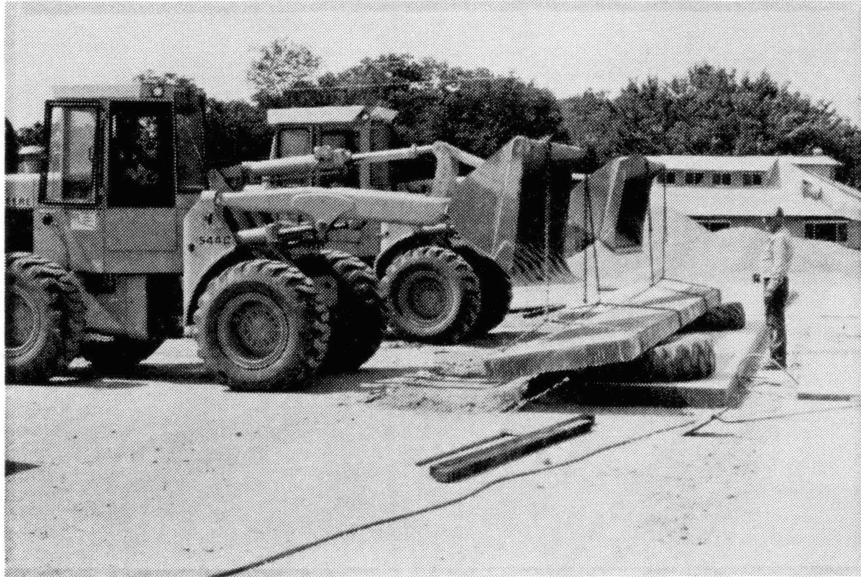
Figure 27. Two Front End Loaders Lifting Panel in a Horizontal Position
