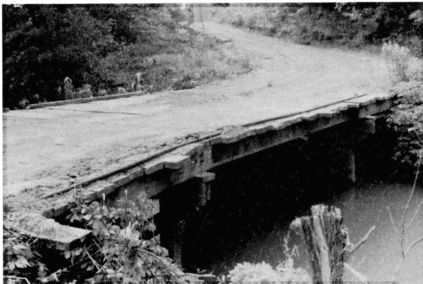
Figure 12. Existing Bridge Viewed from the South
