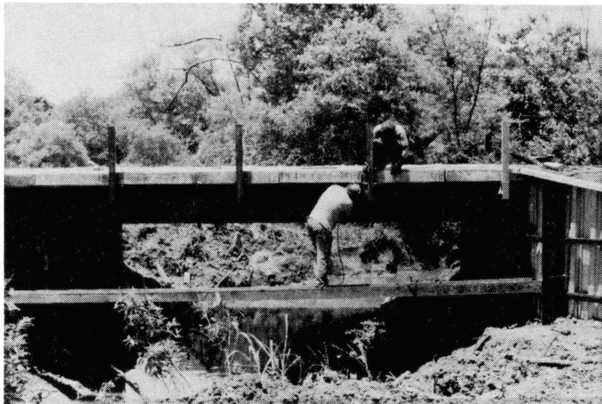
Figure 43. Connection of Traffic Rails
