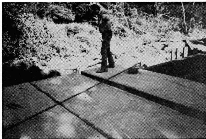
Figure 34. Panel Alignment Utilizing Hook with Chain
