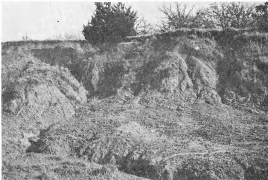
Figure 3.4. The Eroded Slope from Which Sample 203 was Obtained
