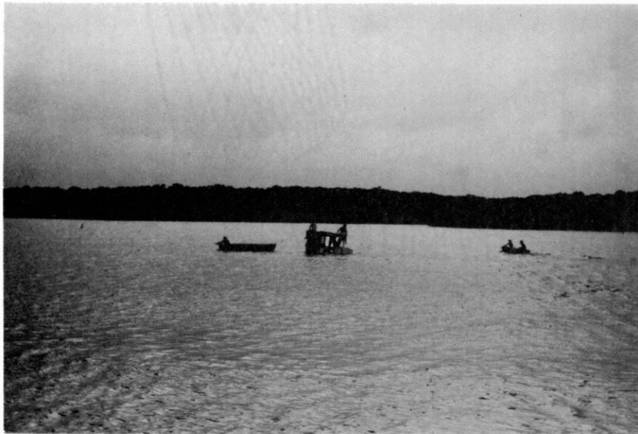
Figure 18. Pump Being Towed Into Position
