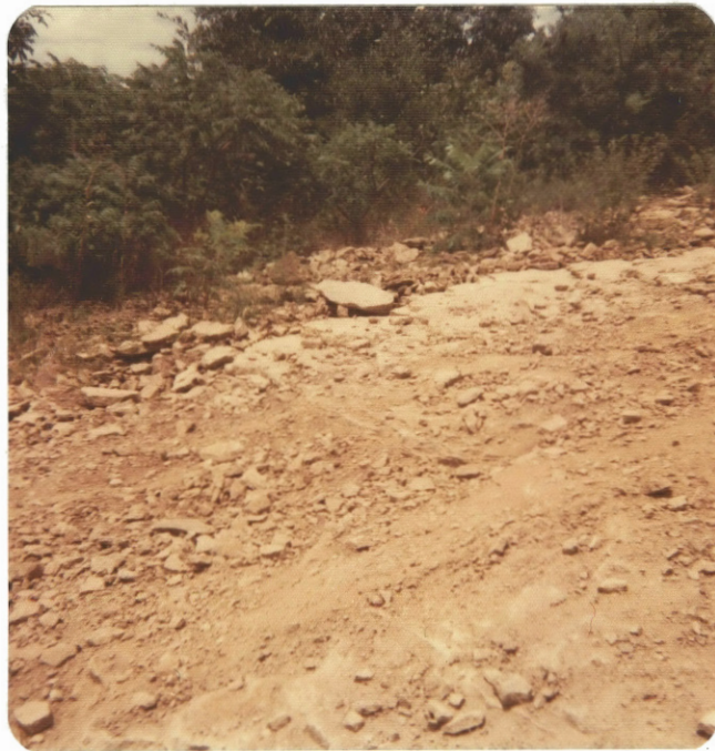
Figure 7.--Example of a deteriorating road on an outcrop of sandstone.
