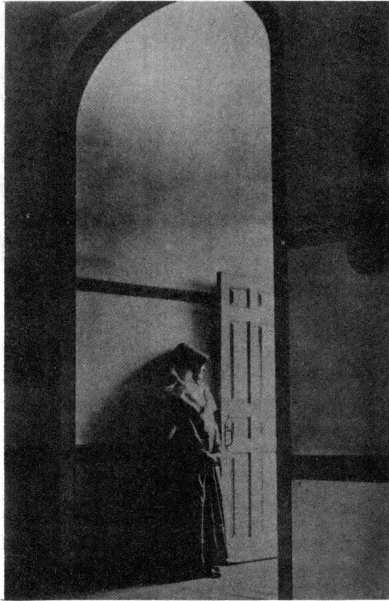
Figure 22. Arched Doorway, Pleasant Hill
