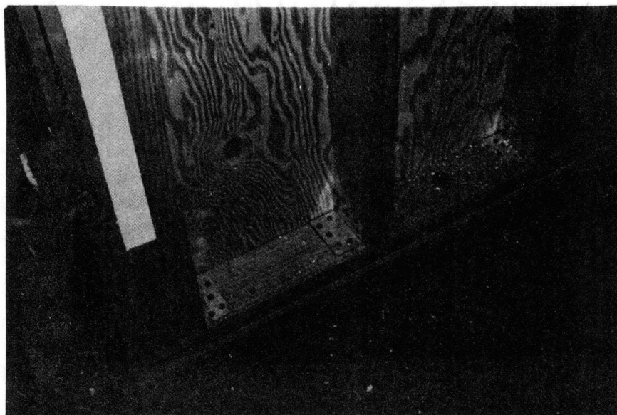
Figure 5. Close-Up of Angle Braces
