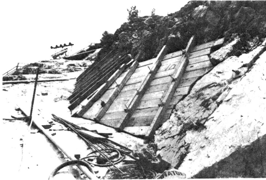
(a) Formwork for Lean-Mix Concrete Placement.
