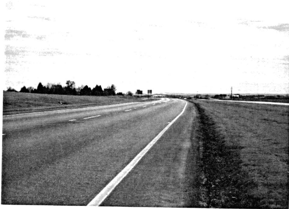
Figure 3.2. Photographs Taken at the Site
