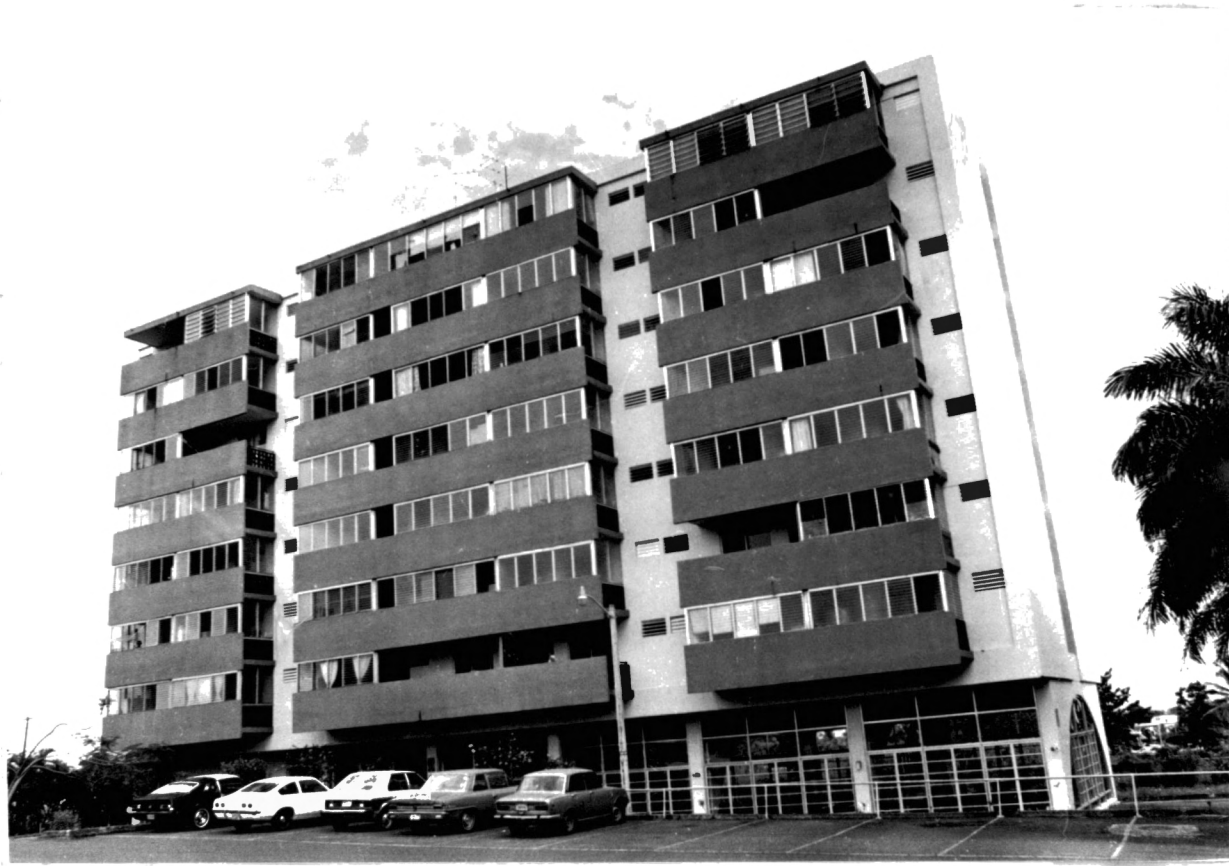
a) Front view of Building
