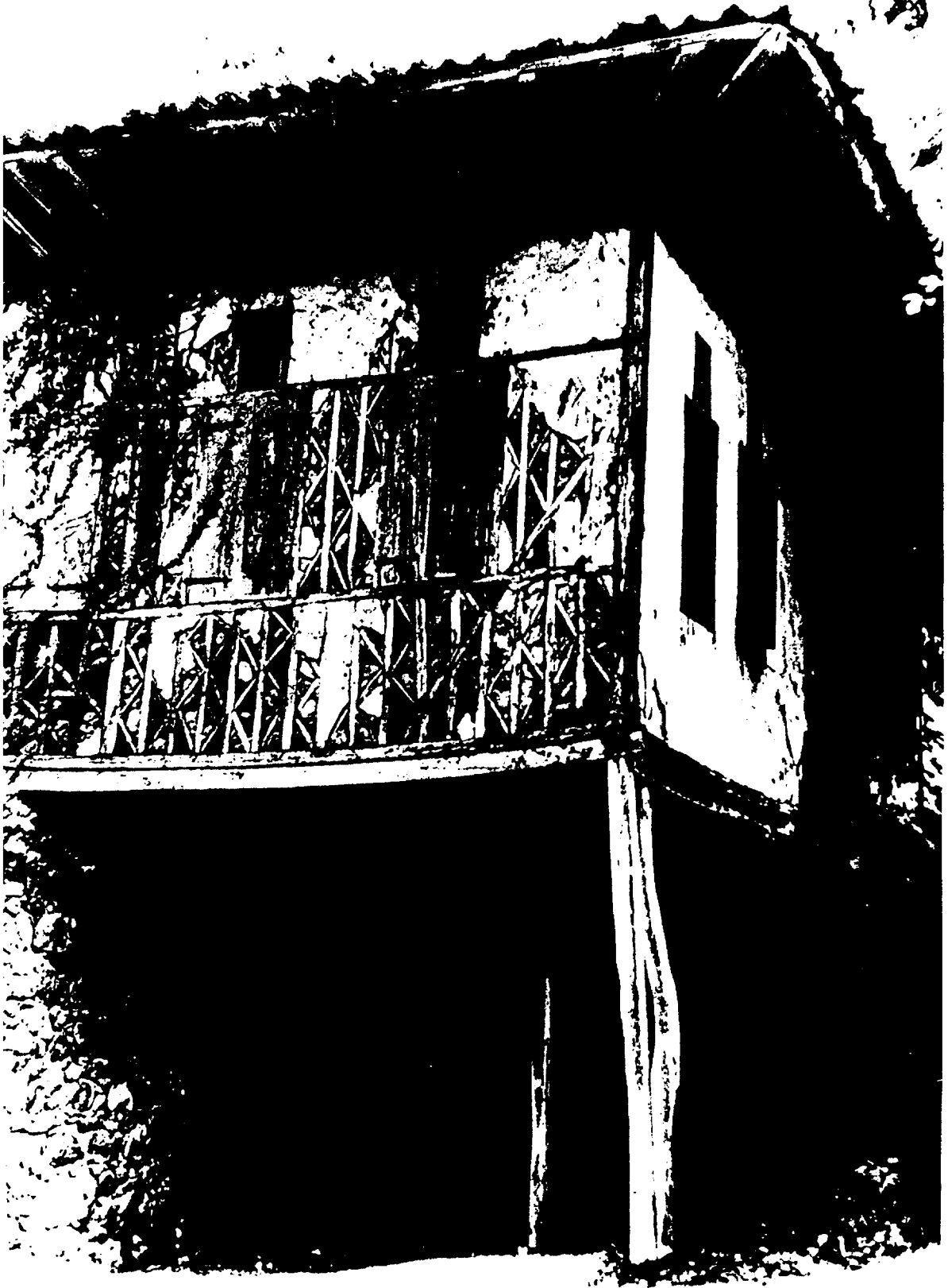
(fig 15) An example of the middle floor resting on wooden pillars. In most cases the middle floor rests on garden walls.
