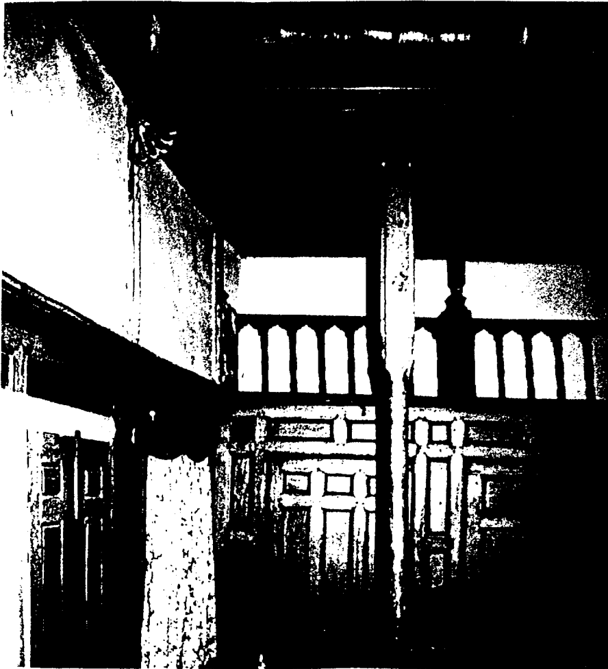
(fig 28) The floor of the iwan is usually raised above that of the hall. In older houses, the iwan may have wooden pillars.
