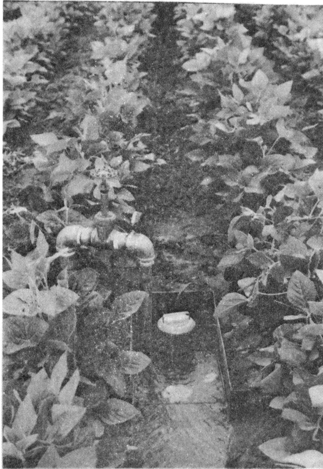
Figure 15. Tailwater Sump and Sump Pump in Place
